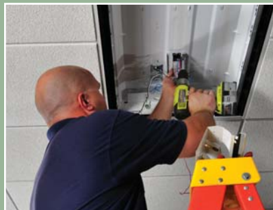
2. Secure Ballast and Socket Tracks.
