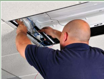
1. Install the Socket Track Flange.
