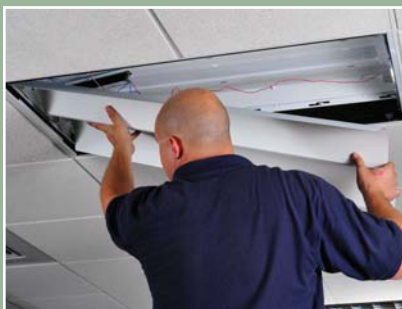
4. Insert Reflector and attach to Socket Tracks (install lamps).
