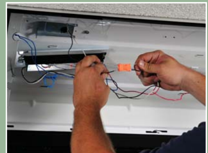
3. Attach Supply Wires to Quick Disconnect.
