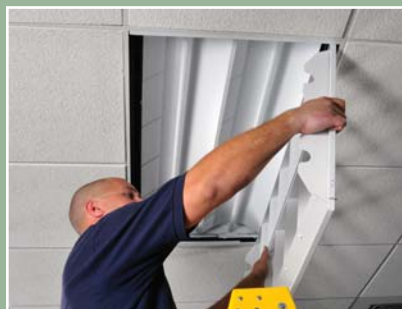
5. Position Louver Hinges into Existing Slots.
