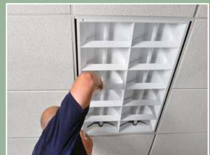
6. Secure Louver by engaging Spring Latches.
