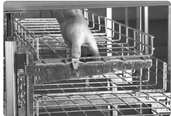
Step 4. Install basket and hold down clips.
