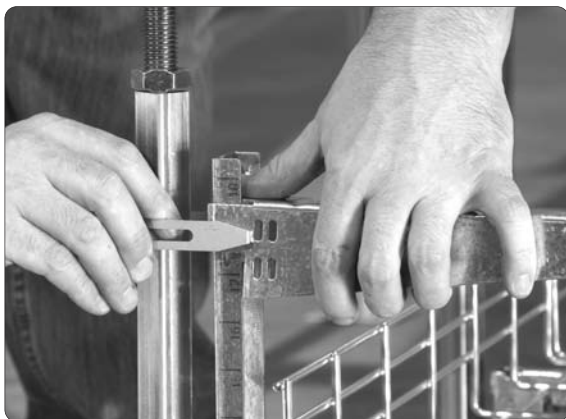
Step 5 (Optional). If desired, install pedestal clips.
