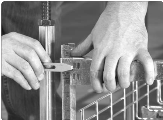
Step 5 (Optional). If desired, install pedestal clips.
