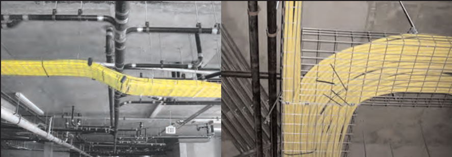
Wire basket installation provides extreme flexibility.
