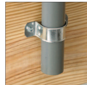
Running CPVC pipe vertically
