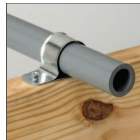
Running CPVC pipe perpendicular across top of beam
