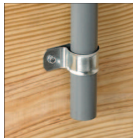
Running CPVC pipe vertically
