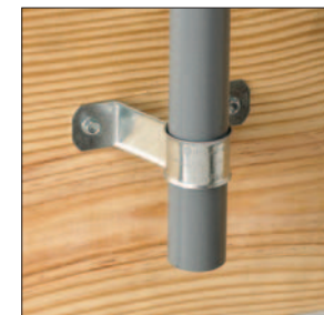
Running CPVC pipe vertically
